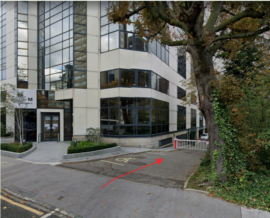
SYDENHAM ROAD ENTRANCE AND VEHICLE RAMP
